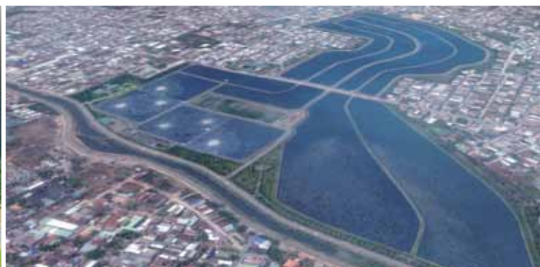
Station d'épuration, 200 000 EH (Ho Chi Minh City, Vietnam)
